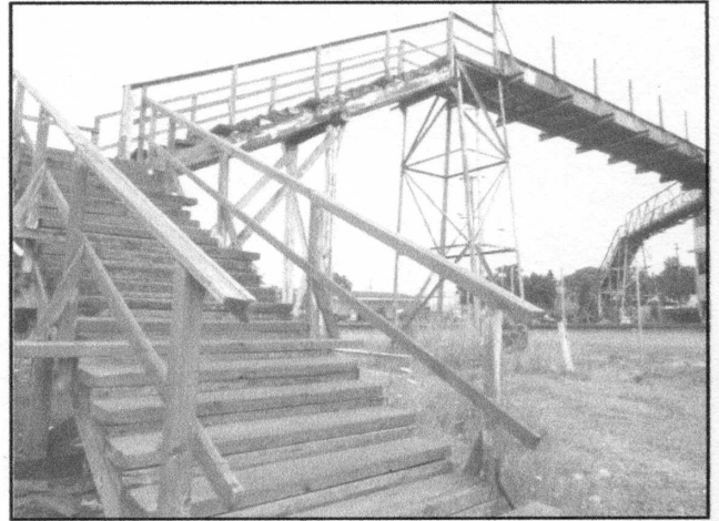
Existing bridge over railroad tracks at the end of Lafayette St.
